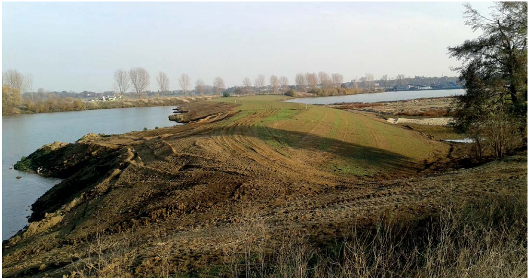
Eind 2018 was de nieuwe centrale dam gereed.
